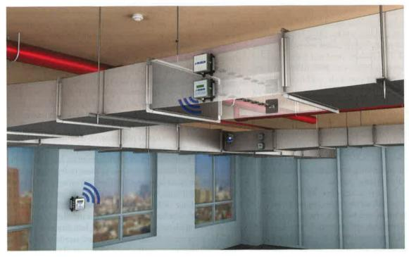
>> Air measurement stations can be installed as part of the ductwork so the station and its placement can be pre-determined.
