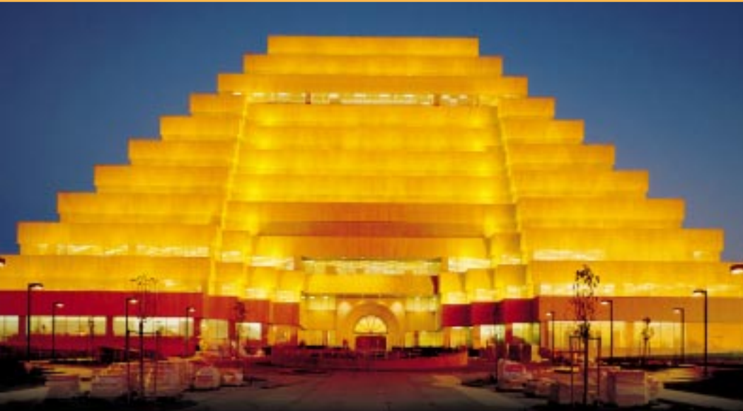
The Money Store Administrative Building, West Sacramento, CA
