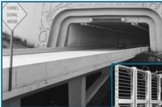
Ruskin supplied CD80 series tunnel dampers to provide smoke control and fan isolation to Seattle Washington's 23rd street automotive tunnel.
