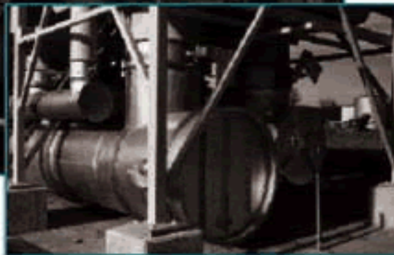
Model CDR195 dampers installed on a Model 5400-5-98-95 US Filter/Huntington Energy Systems Regenerative Thermal Oxidizer
