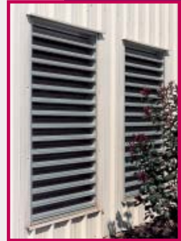
Wal-Mart Distribution Center, Lauren, SC
