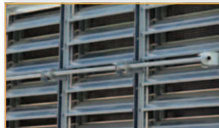
Top view – Ruskin’s high performance ELF6375DX louver finished with a 2-Coat 70% Kynar that matches the aesthetics of the building siding. Bottom view – Ruskin CD36 damper incorporating special spacing to fit around already constructed building structure.
