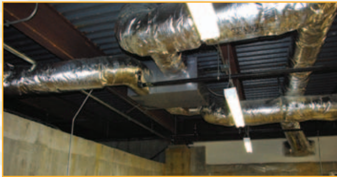
The low profile of the MV 750 makes for easy installation in tight spaces above the ceiling.
