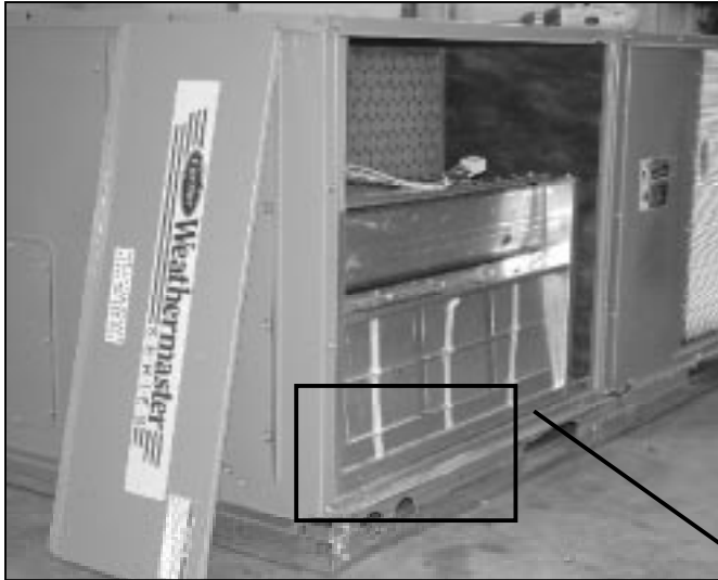
Front flange of economizer sits in front of rooftop mating flange as shown
