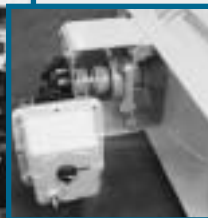
Ruskin damper model CDRI92 can be easily adapted to provide tight shut-off in large openings. This 10' x 10' (3.048 M x 3.048 M) CDRI92 equipped with full circumference silicone blade seals meet leakage of 14 cfm (.39648M 3 ) total per section. Electric 2 position actuators were installed with right angle gear boxes and direct coupled to a 3" (76.2 MM) O.D. extended damper output shaft.
