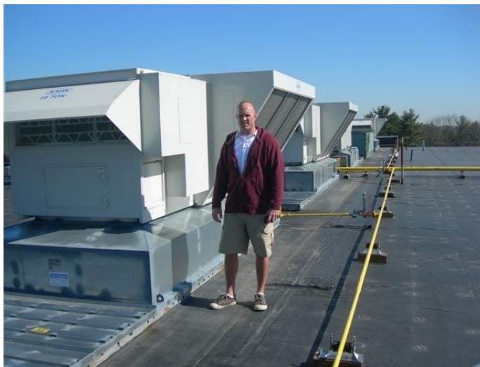
Custodian Tim Fournier comments there is no added maintenance for the energy recovery wheels.
