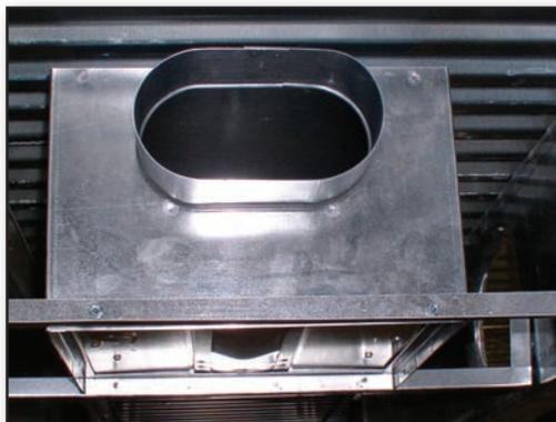
CFD7 installs with angles attached to the sides of the joist. Angles may be factory or field supplied.
